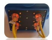
2. If applicable, turn on the stand-alone fans. Then turn on the fan on the heater (the green switch) and then the heater (the red switch). The heater is preset to 75°F. This should be sufficient to heat your room. If you need more heat, press the "Set" button and adjust the thermostat accordingly. The heater is programed to have a maximum thermostat setting of 105°.F
